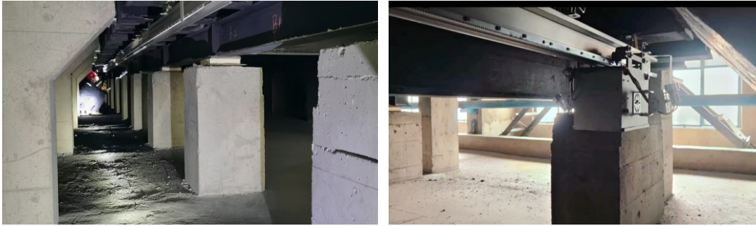
Figure 6. Synchronized measurement by manual and inspection robots.
